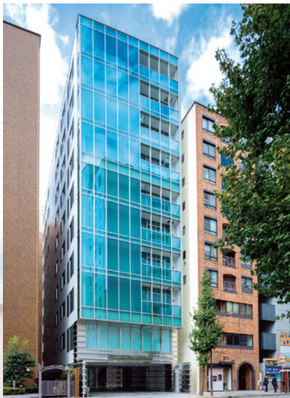
TOSHIN HONMACHI BUILDING
